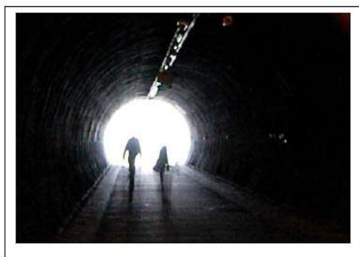
Figure 2. Light at the ‘End of the Tunnel’.
